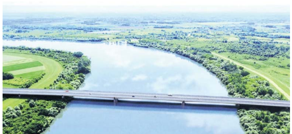
Design drawing of the future bridge over the River Sava in Svilaj, Bosnia and Herzegovina
