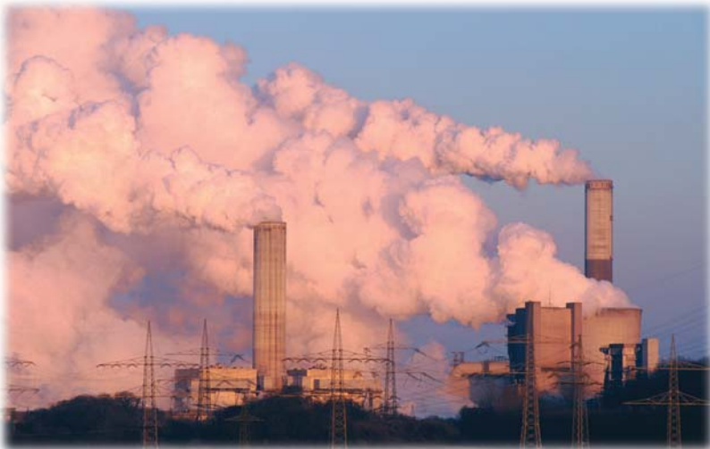
Burning coal to produce electricity is particularly harmful to the climate.
