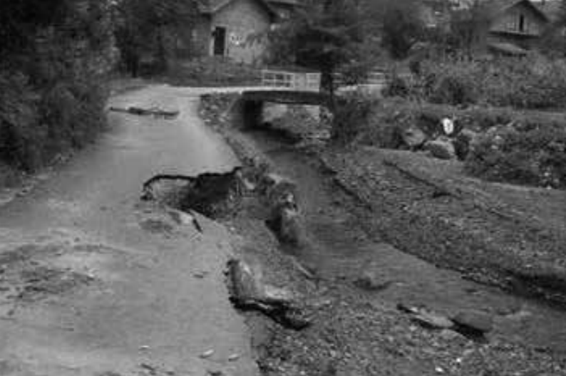
Teslić: Local road in Rajševo LC (before and after rehabilitation)
