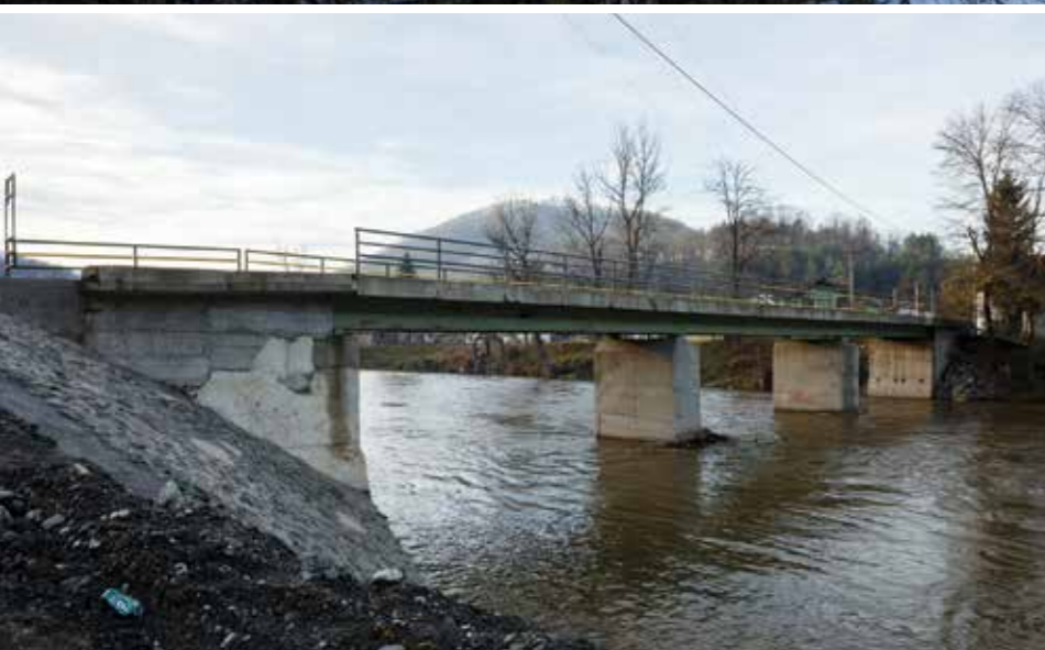
Zavidovići: Rehabilitated bridge in Brezik LC
