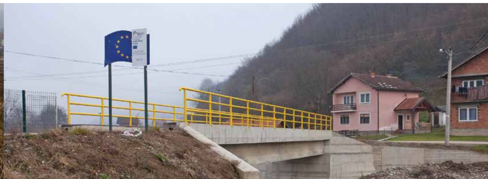
Milići: Rehabilitated Dubnički bridge on the river Jadar
