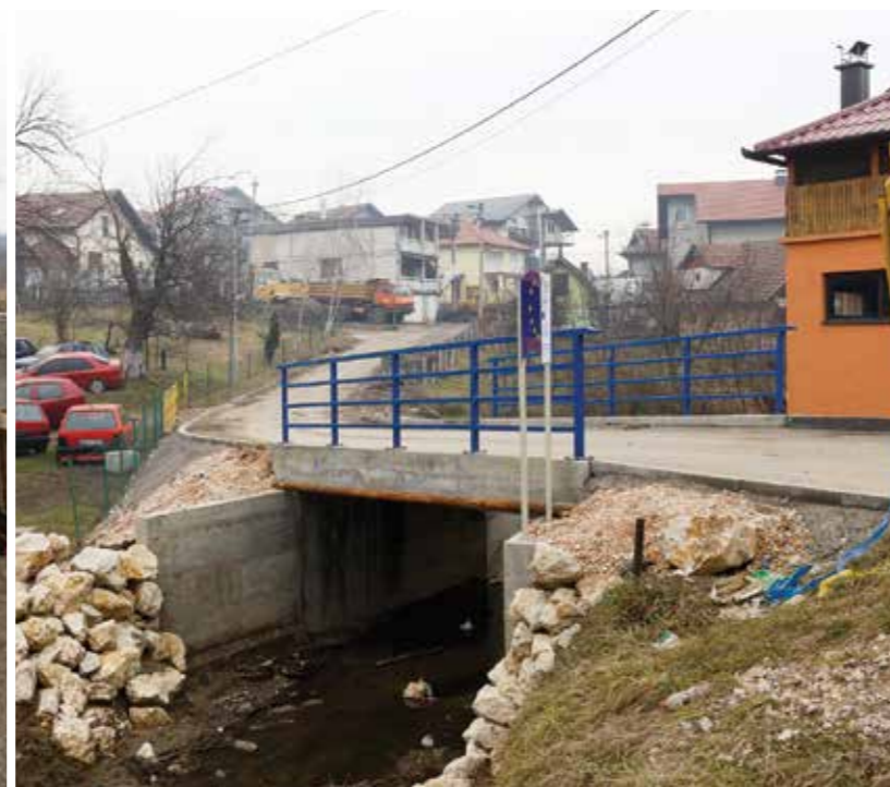
Tuzla: Rehabilitated Solana bridge on Moluška river
