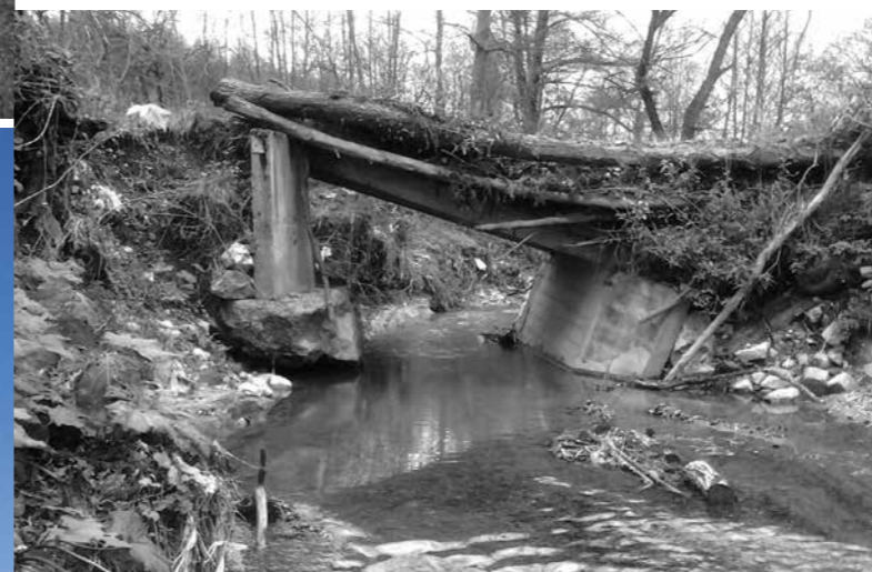
Kalesija: Bridge in Kikači LC (before and after rehabilitation)
