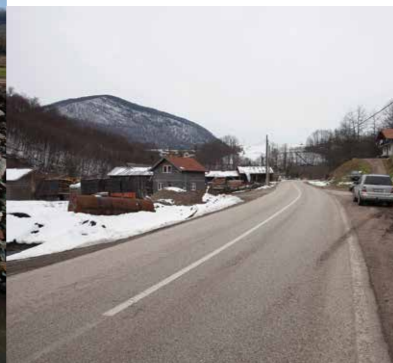
Kladanj: Rehabilitated local road in Gazdići
