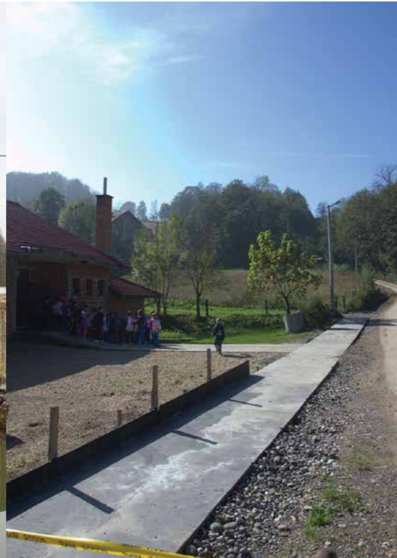
Doboj-East: Rehabilitation of local road in Klokočnica LC
