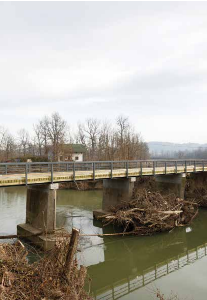
Derventa: Rehabilitated bridge in Derventa
