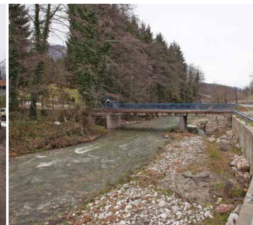
Kladanj: Rehabilitated bridge
