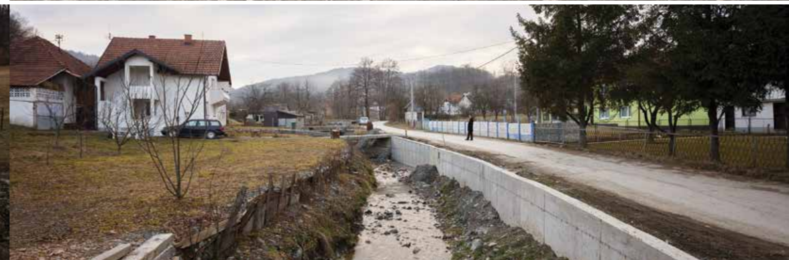
Rehabilitated road infrastructure in the area of Banovići
