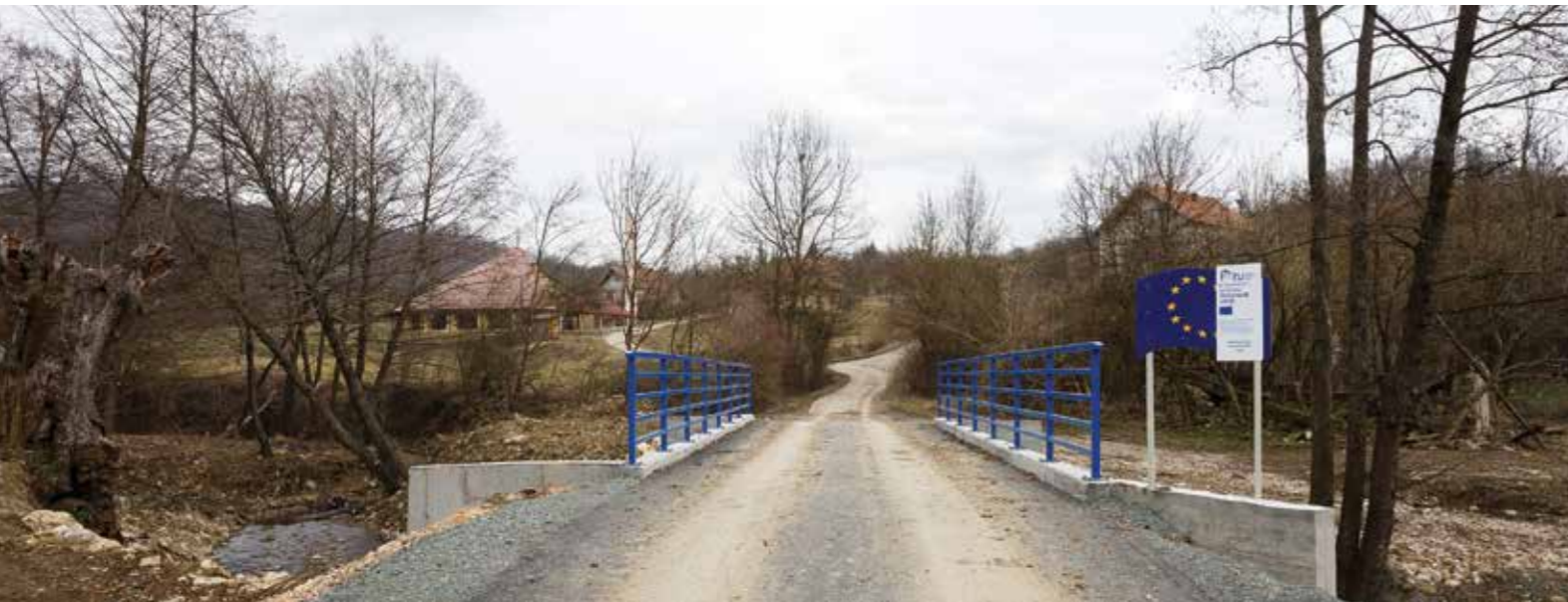
Tuzla: Rehabilitated Dokanj bridge
