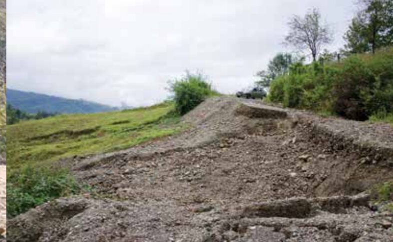
Kotor Varoš: Rehabilitation of Garići local road in Maslovare LC
