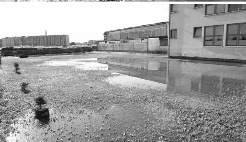
Derventa: Nikola Tesla Elementary School (before and after rehabilitation)
