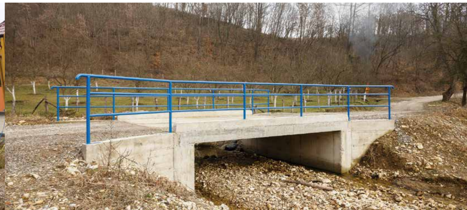
Vukosavlje: Rehabilitated bridge in Gnonica
