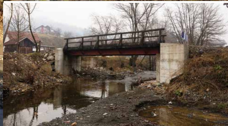
Maglaj: Rehabilitated bridge Megara Jablanica
