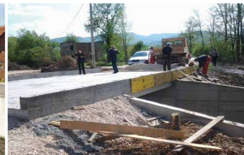
Živnice: Rehabilitation of the bridge on the river Krivača
