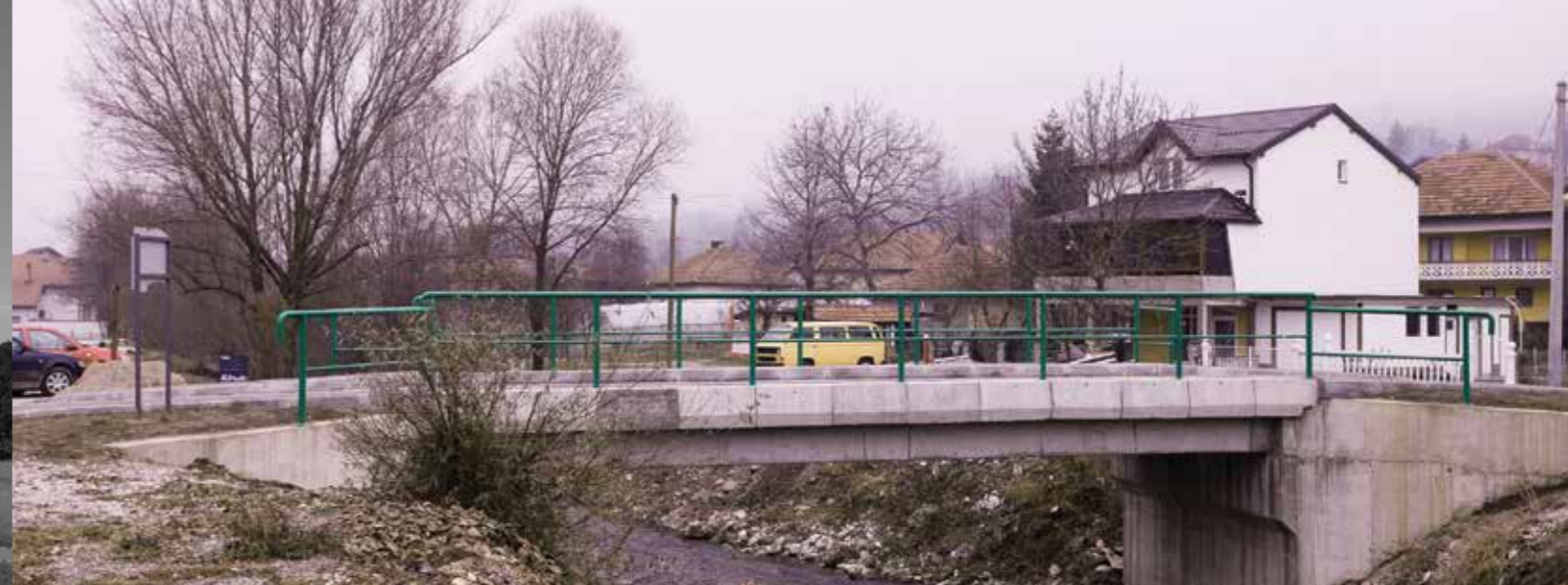
Kakanj: Rehabilitated Zgošća bridge
