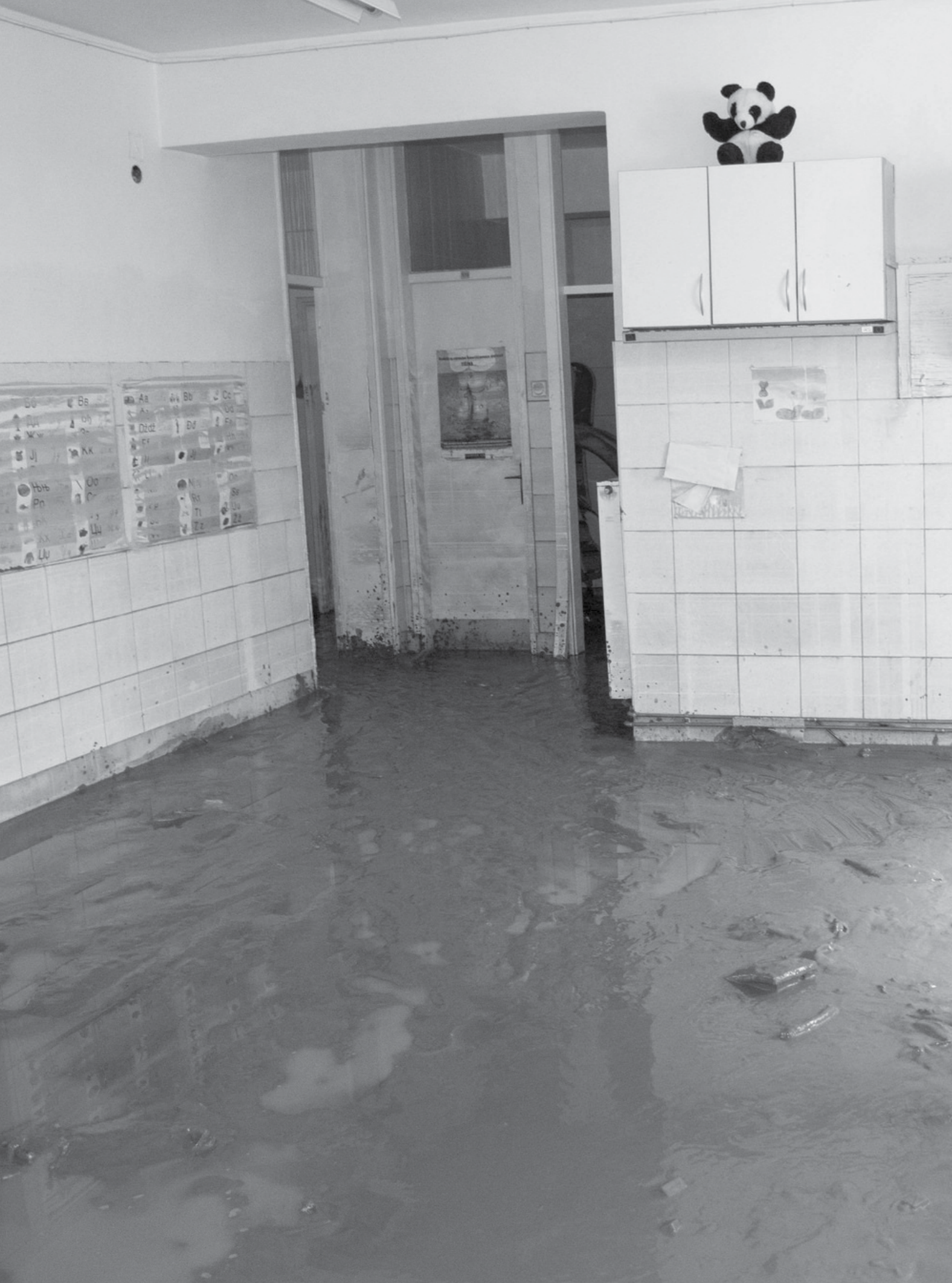
Health Care Centre Doboj (before and after rehabilitation)
