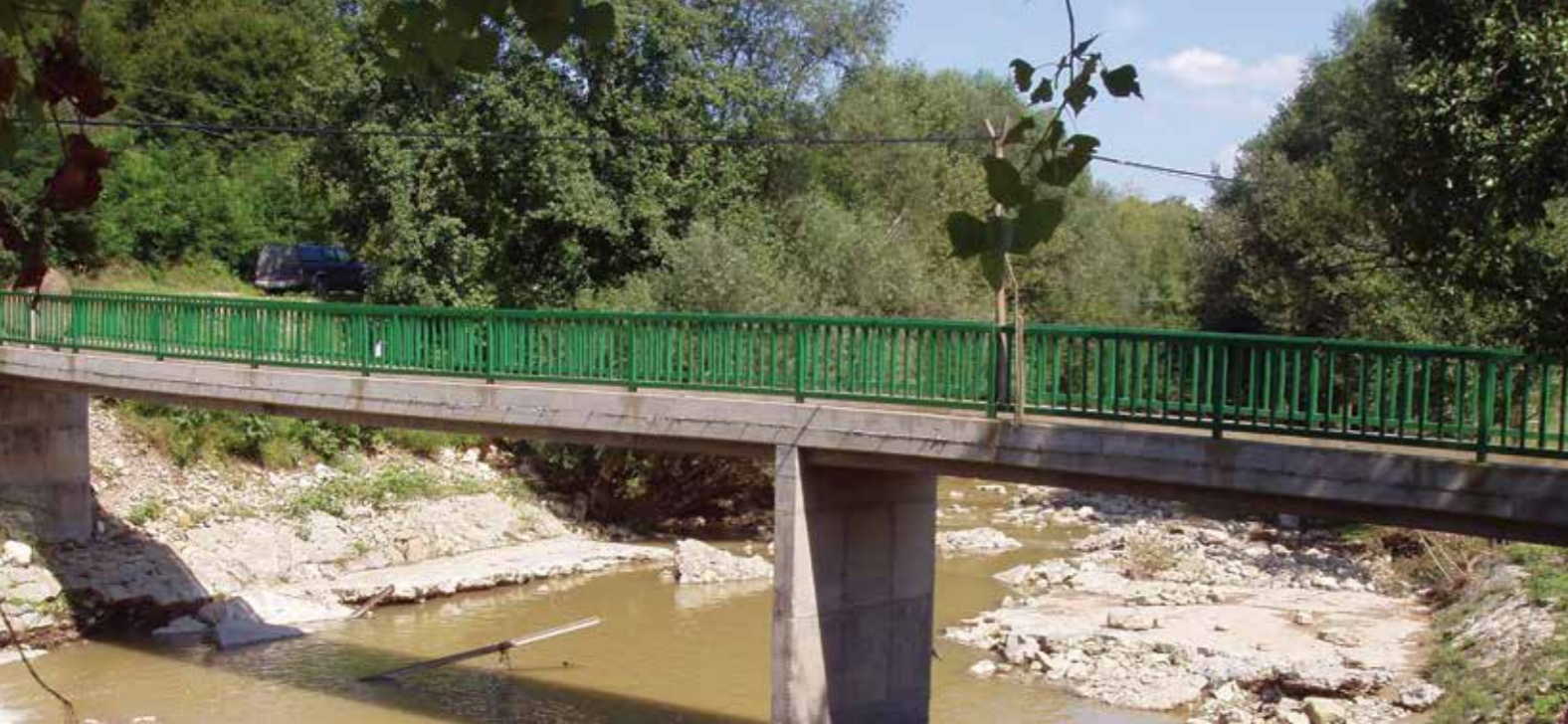
Čelić: Rehabilitated bridge in Brana, Vražići
