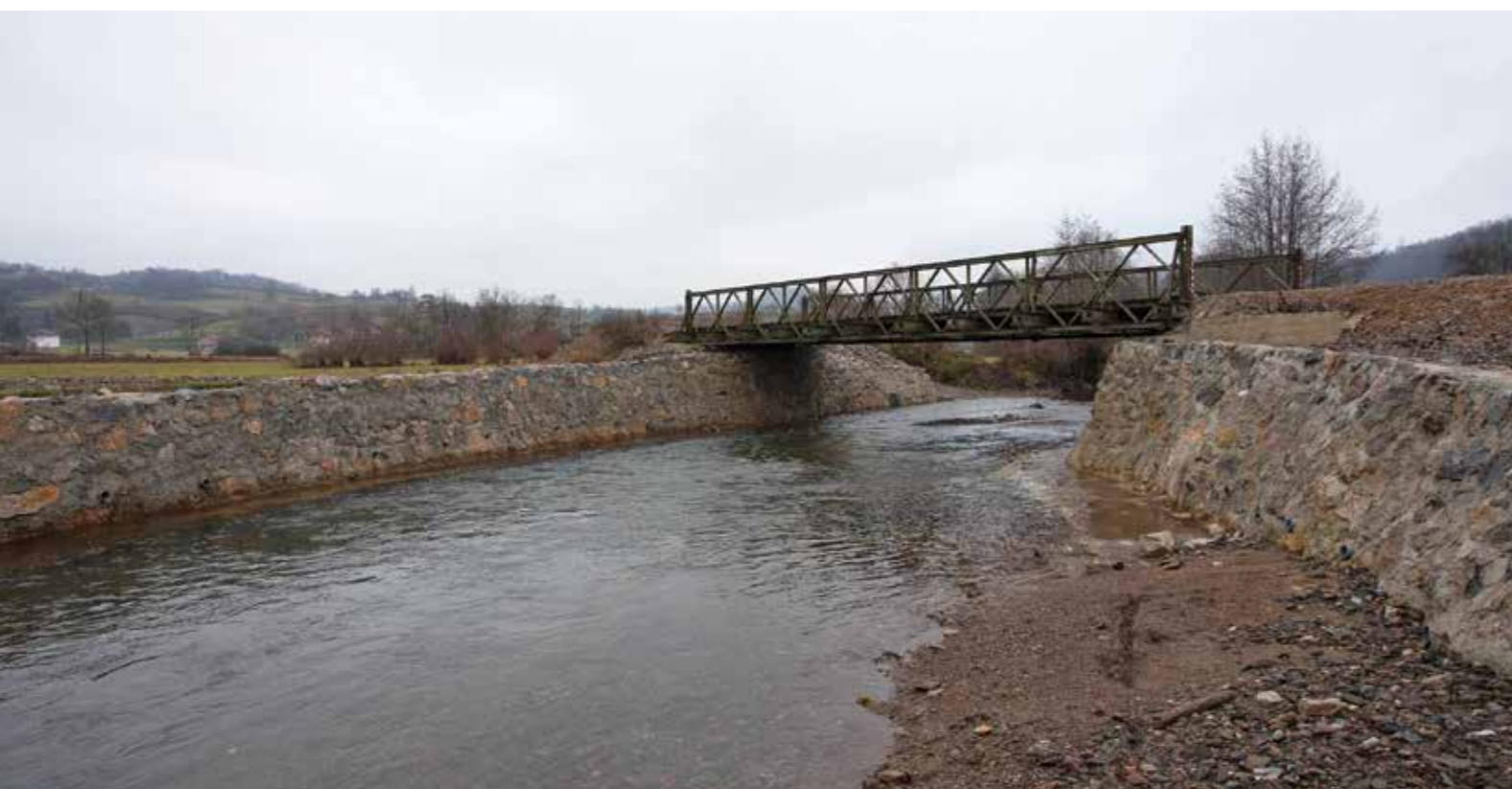
Novi Grad: Rehabilitated bridge in Jagodnjak LC, river Japra
