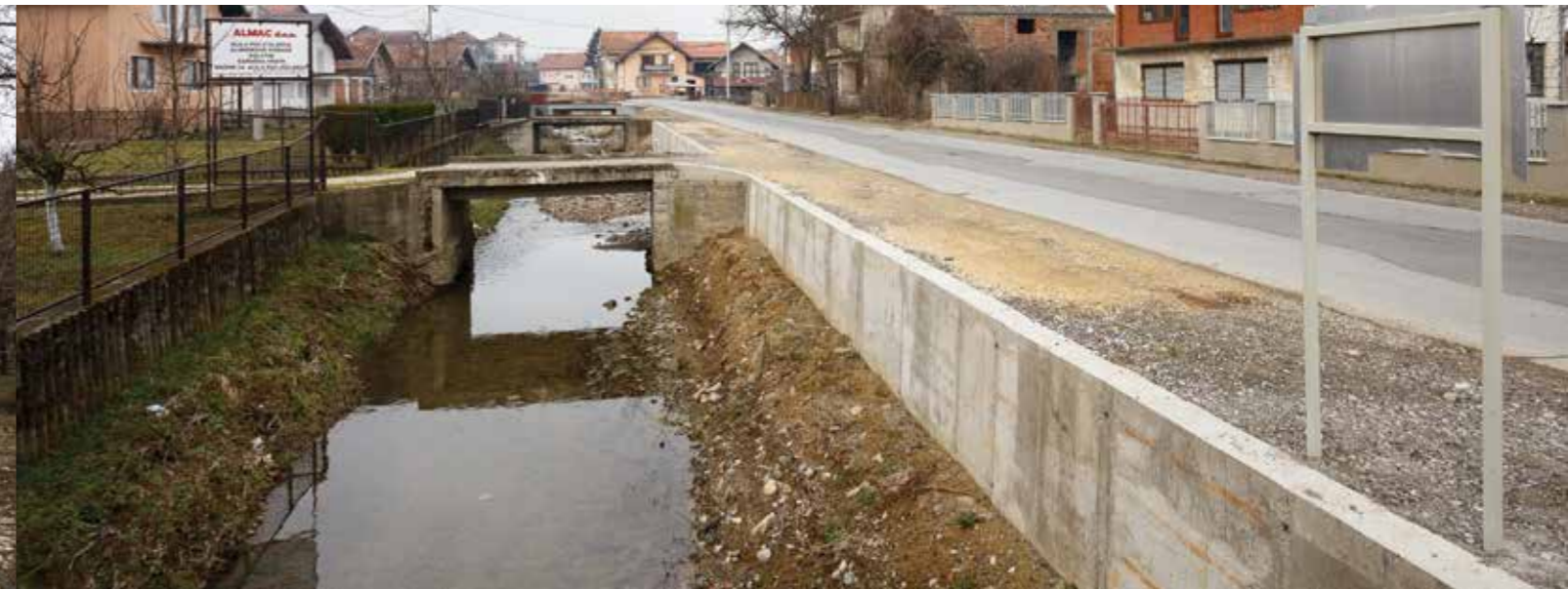
Vukosavlje: Rehabilitated retaining wall on Jakišnica river
