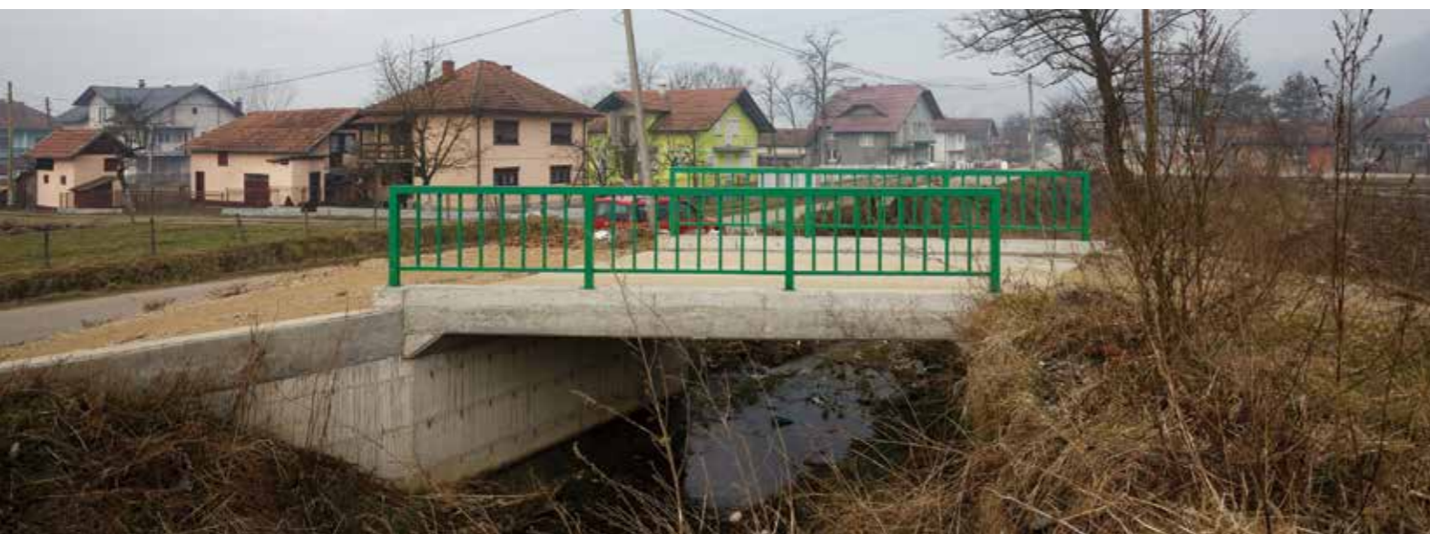
Lukavac: Rehabilitated bridge in Gnojnica LC
