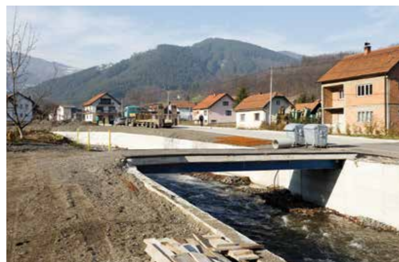
Žepče: Rehabilitation of bridge in Papratnica LC
