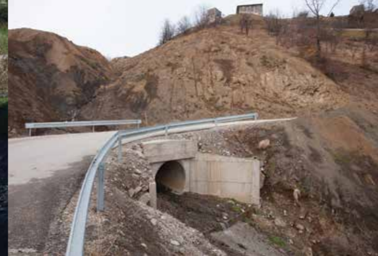
Vareš: Rehabilitated culvert
