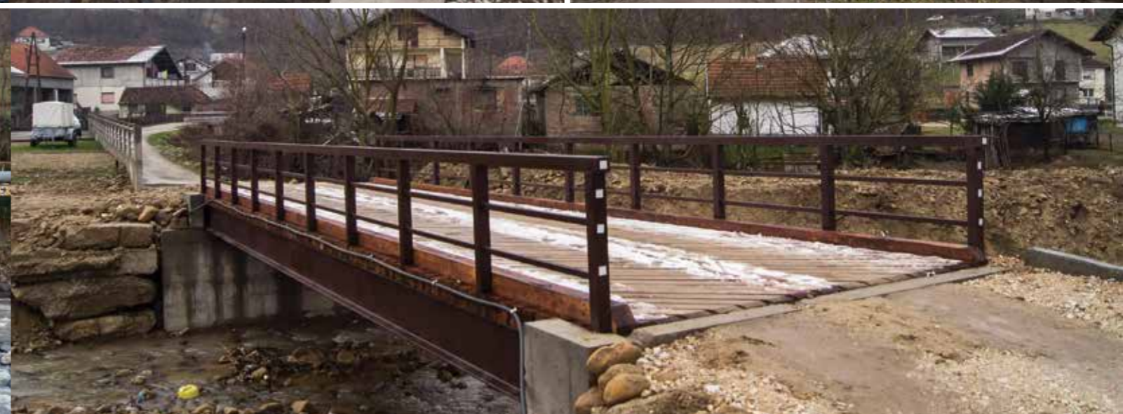
Zvornik: Rehabilitated Jasenice bridge
