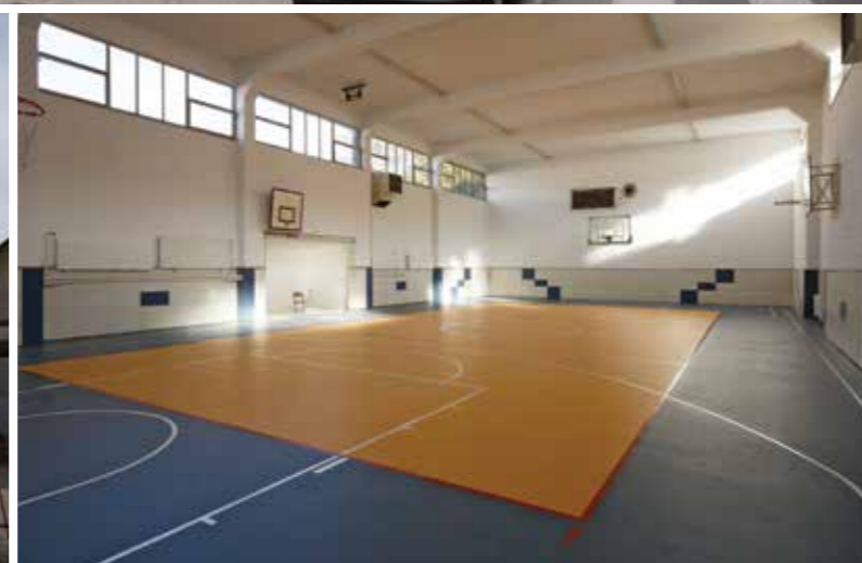
Žepče: Rehabilitated Žepče Elementary School (school gymnasium)
