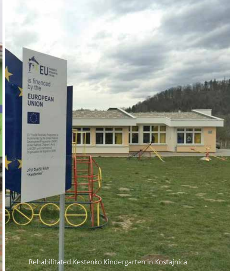
Rehabilitated kindergarten in Domaljevac – Šamac
