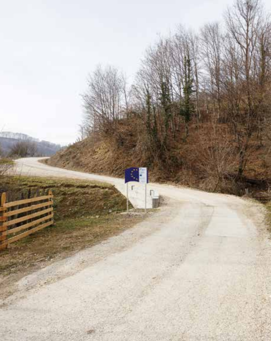
Modriča: Rehabilitated local road
