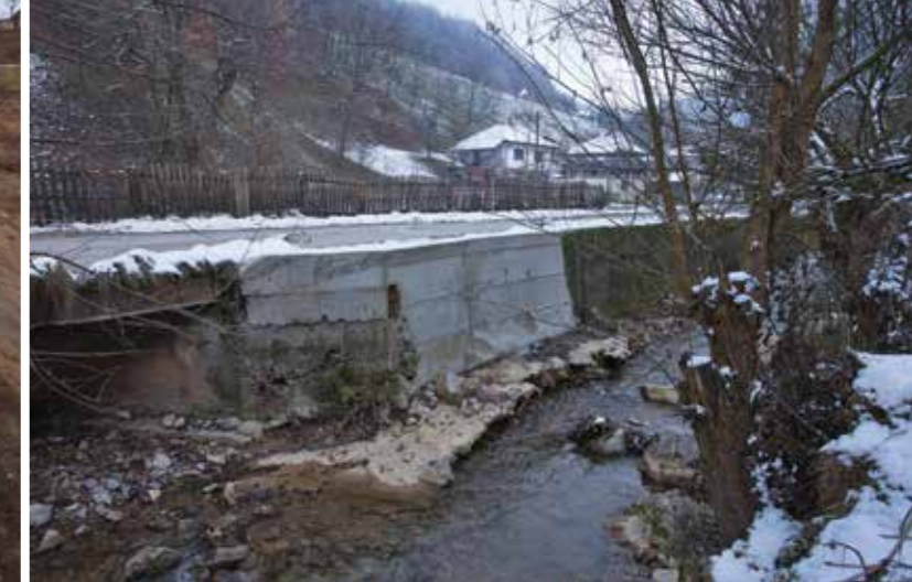
Vareš: Rehabilitated culvert
