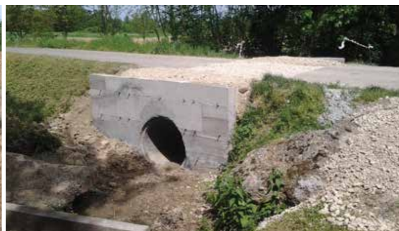
Pelagićevo: Rehabilitated culvert in Kesterovići
