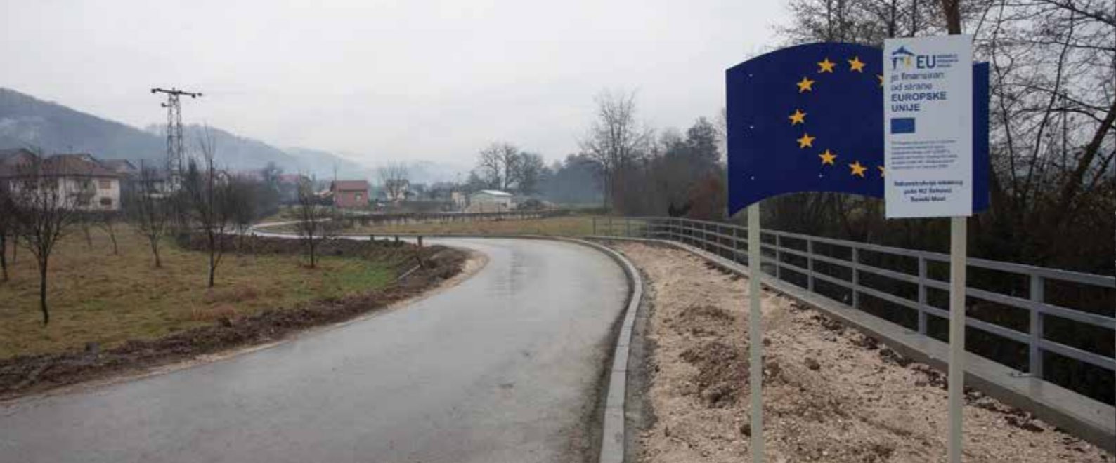
Sanski Most: Rehabilitated local road in Šehovci LC
