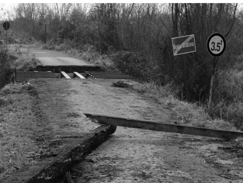
Šamac: Tolisa bridge (before and after rehabilitation)
