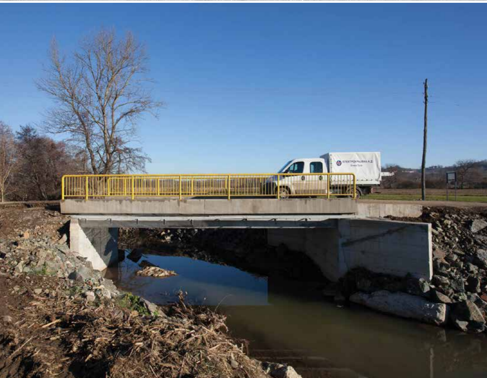
Gradiška: Lubina bridge, Turijak (before and after rehabilitation)
