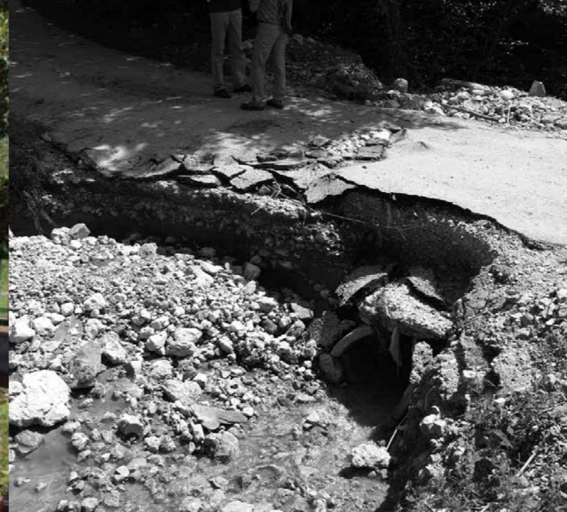
Doboj-East: Culvert (before and after rehabilitation)
