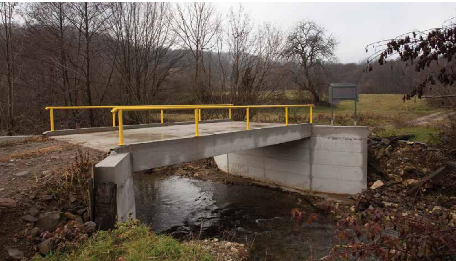
Kostajnica: Rehabilitated bridge in Dženadije LC
