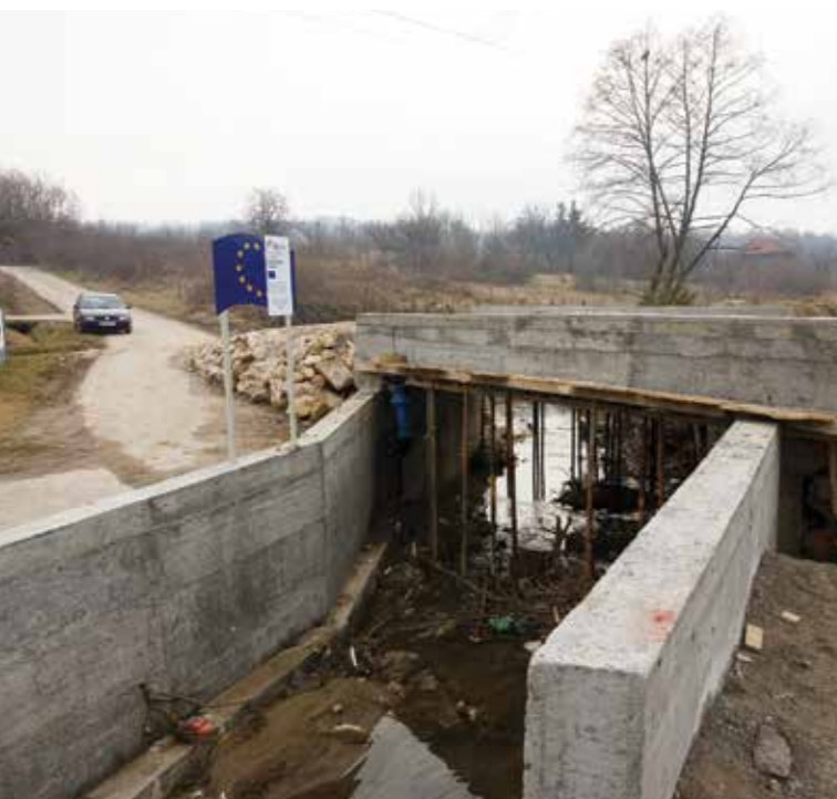
Tuzla: Rehabilitated Mazići bridge, Dobrnja
