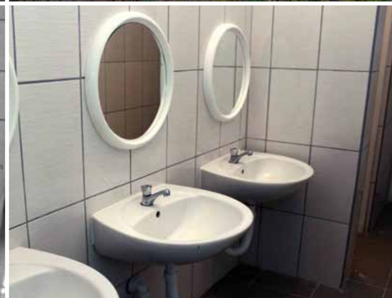
Odžak: Vladimir Nazor Elementary School, Prud, (before and after rehabilitation)
