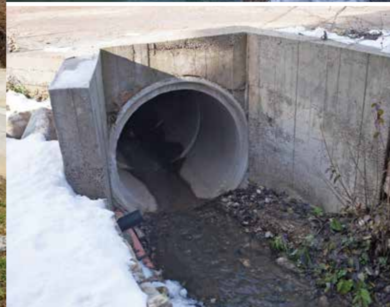
Olovo: Rehabilitated culvert
