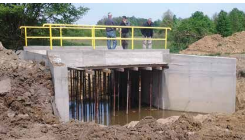
Pelagićevo: Briježnica bridge rehabilitation
