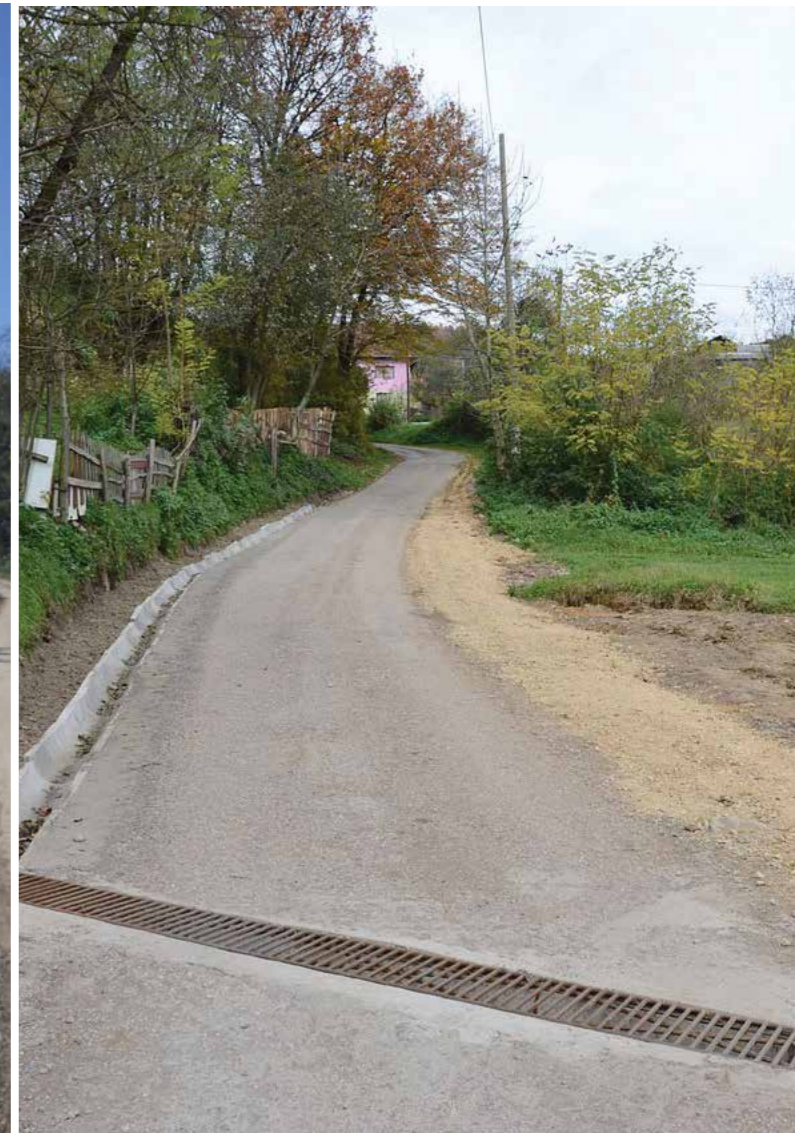
Doboj-East: Rehabilitated water drain
