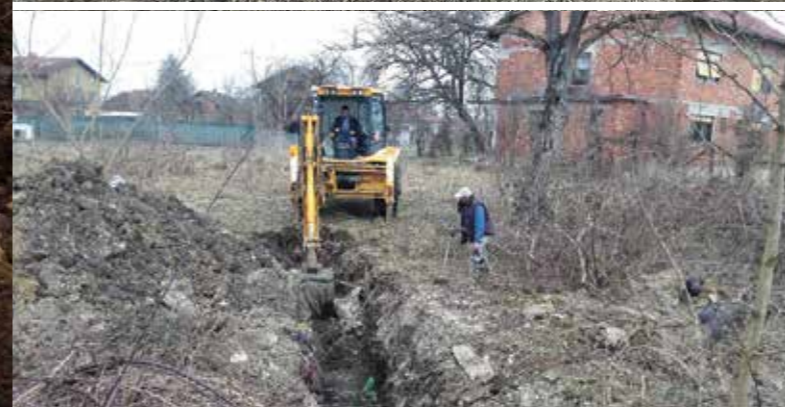
Kozarska Dubica: Rehabilitation of sewer
