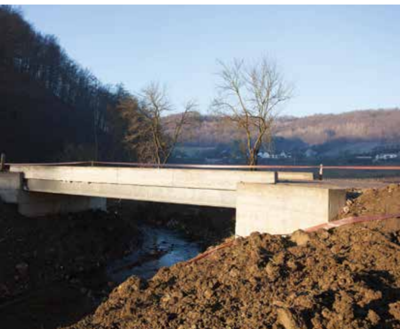
Srbac: Rehabilitated Korovi bridge
