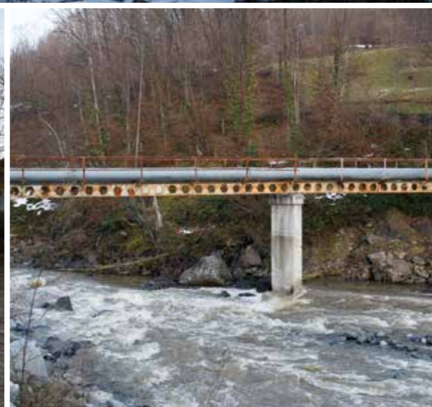
Zavidovići: Rehabilitation of the main water supply system
