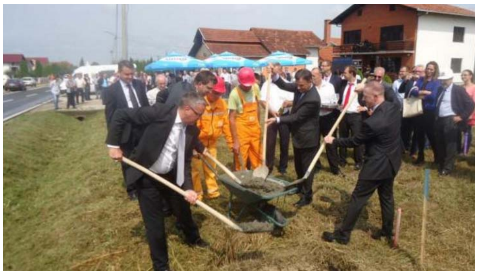
Laying the foundation stone of the Brcko bypass (September 2015). Works are ongoing. The EU has contributed with a €0.5 million project implementation support grant.
